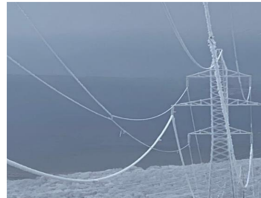
GSE operated EHV/HV lines damaged due to climate hazards
